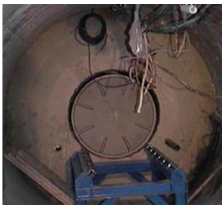
(a) Installation status of heater
